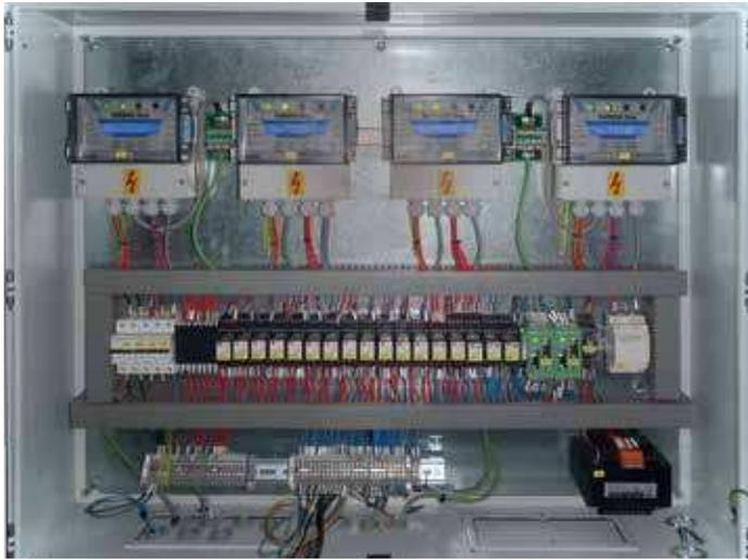
**SIDEOS One** is a programmable and secure module for speed monitoring, fitted with an efficient auto control system which secures the overall operation of the overspeed detection system.
